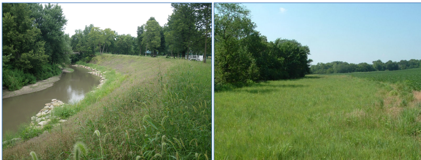
Figure 3. CPs installed in the Delaware River Watershed includes stream bank restoration and riparian buffer protection.
